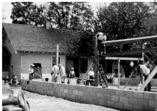
Picture 2. Early Annex construction/
