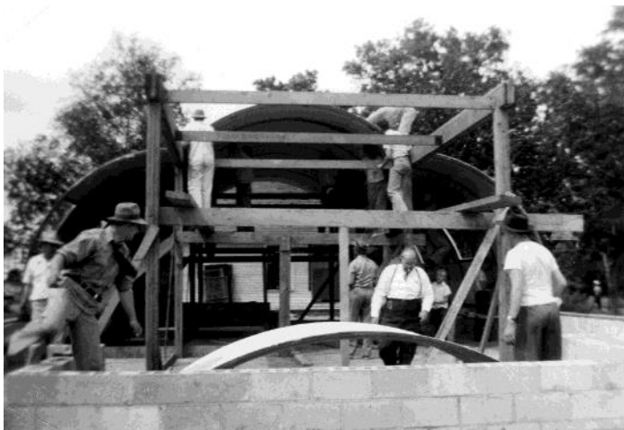
Picture 3. Raising of the Hutment sections.
