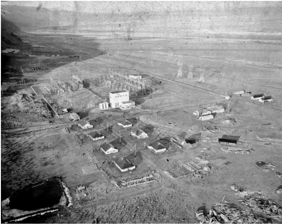
Midway Substation circa late Summer 1942, looking NW. Cottages are in the foreground, and the cluster right of center is presumably the dorm, Post Office, school, etc.
